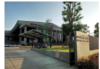
ACTIVE BONDED WAREHOUSE CO., LTD. @LAT KRABANG
