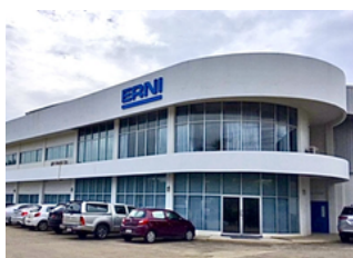
ERNI ELECTRONICS @NORTHERN REGION INDUSTRIAL ESTATE
