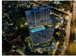
LUMPINI MIX SALES GALLERY @NARATHIWAS - RATCHADA
