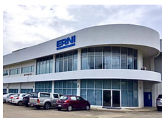
ERNI ELECTRONICS @NORTHERN REGION INDUSTRIAL ESTATE
